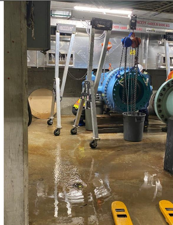
Photo 6: High lift pump pipe gallery showing installation of isolation valve
