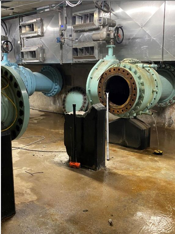
Photo 5: High lift pump pipe gallery showing existing control valve to be removed
