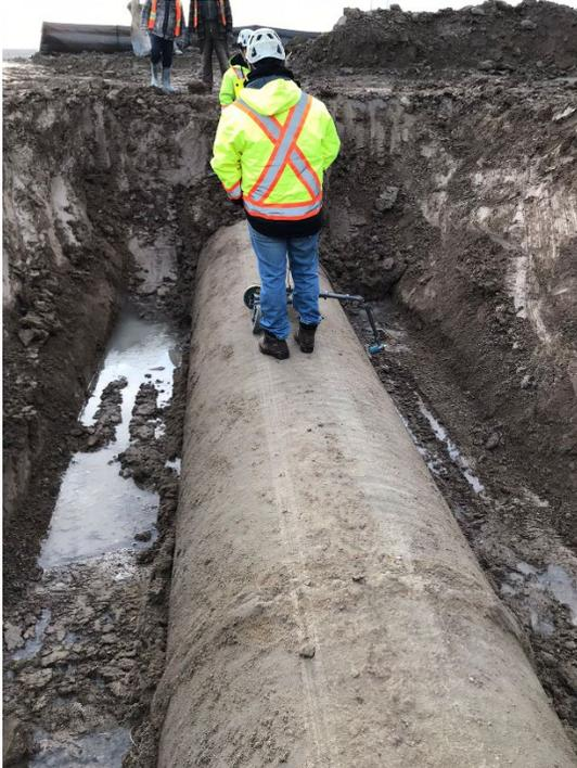
External Electromagnetic Verification of the Pipe
