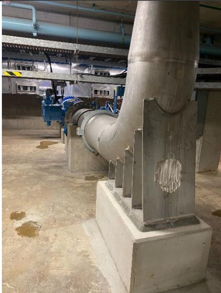
Photo 7: High lift pump pipe gallery showing new high lift pump 5 discharge piping, control valve and isolation valve
