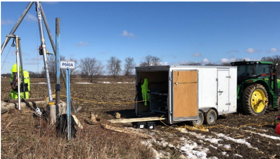
Figure 4d: Elgin 750mm pipeline PureRobotics™ electromagnetic inspection; set up at a pipeline chamber.
