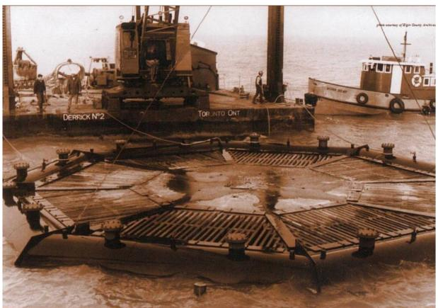
(1966) Positioning the intake structure in Lake Erie before submersion
